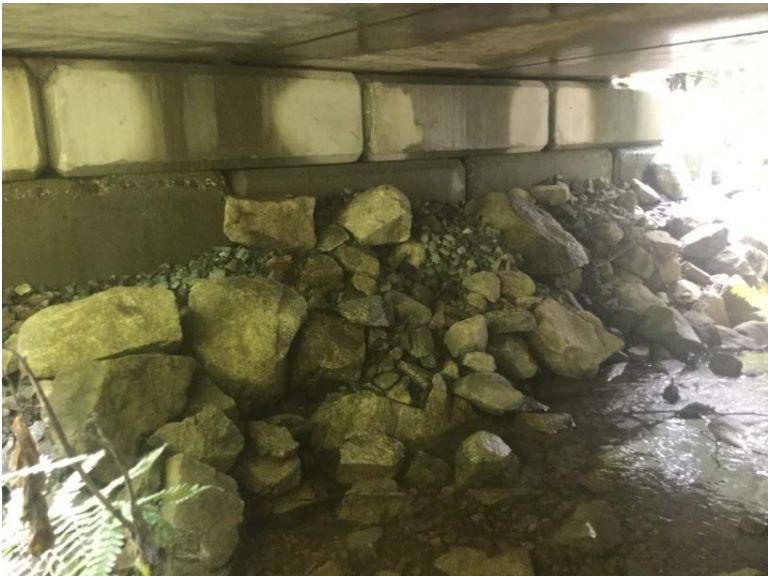
Left Bank Abutment when facing downstream
