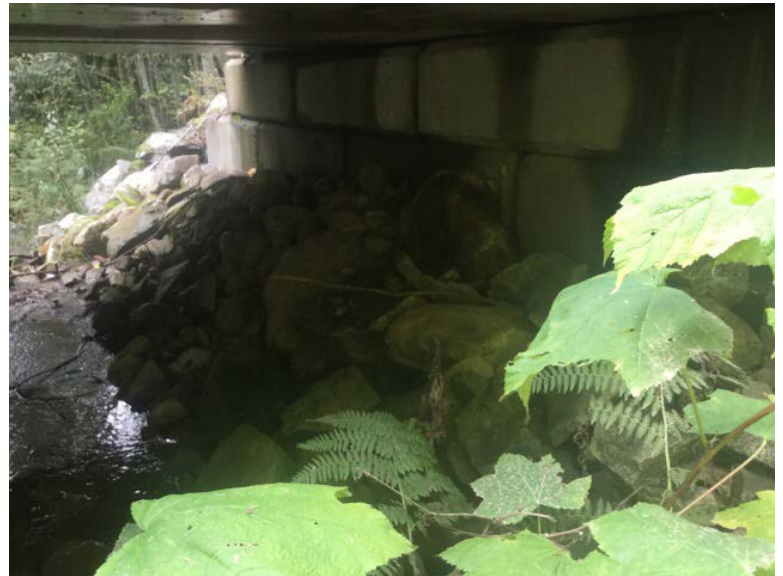
Right Bank Abutment when facing downstream
